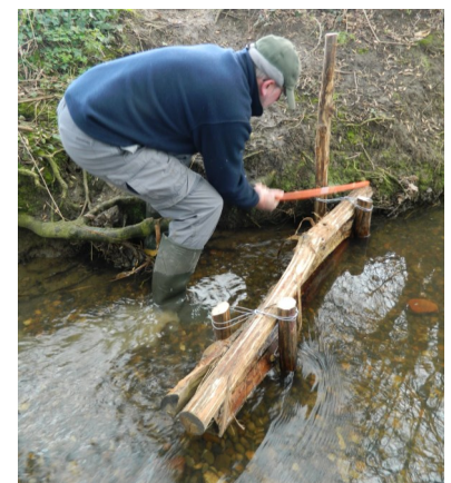
Cutting the wooden pegs to size
