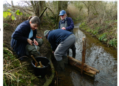
Securing the pegs in place with wire
