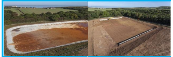
Phase 1 – sludge drying bed
