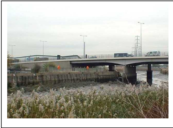
View from the opposite bank before works
