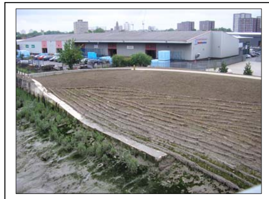
Retreated flood defences post works
