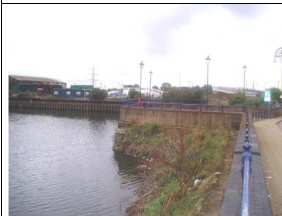
Frontage before terracing work
