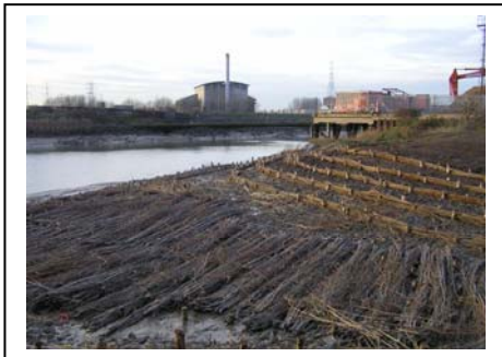
Constructing the inlet
