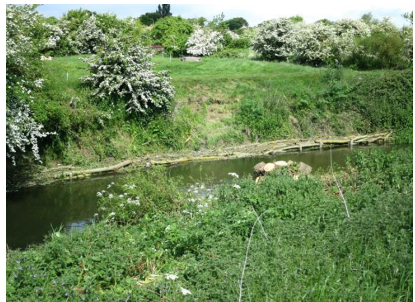
Above - Finished reveted bank
