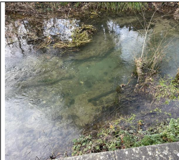
Deep Scour pool between narrowing berms Winter 2022. Credit: EA
