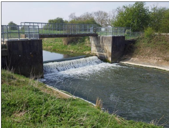
Fig 1. Before – Aubourn Weir showing the drop of around a metre which created a barrier to the passage of fish and eels.
