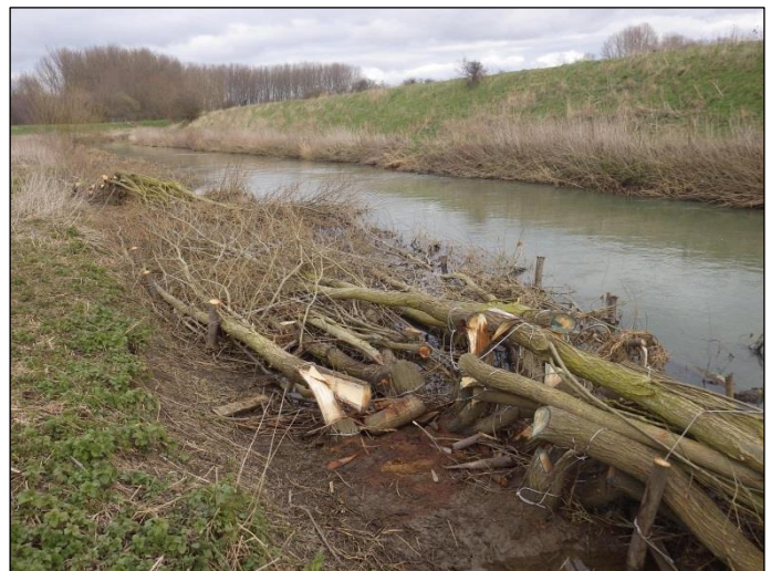
Fig 3 (Before) and Fig 4 (After). Large riverside trees were selectively hinged and secured along the bank and into the water to create valuable instream woody habitat and provide refuges for fish and invertebrates as the river level fluctuates.
