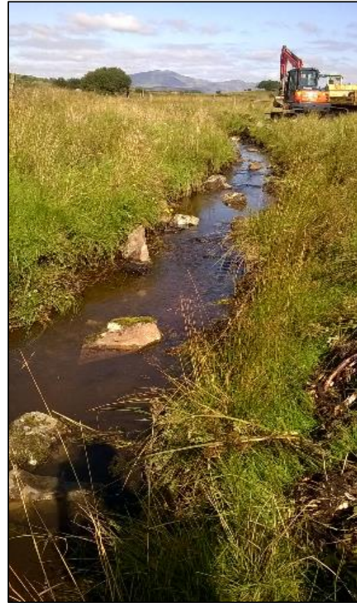
Boulder placement - After
