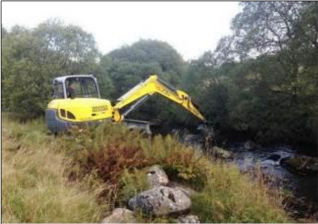
Boulder placement - Before
