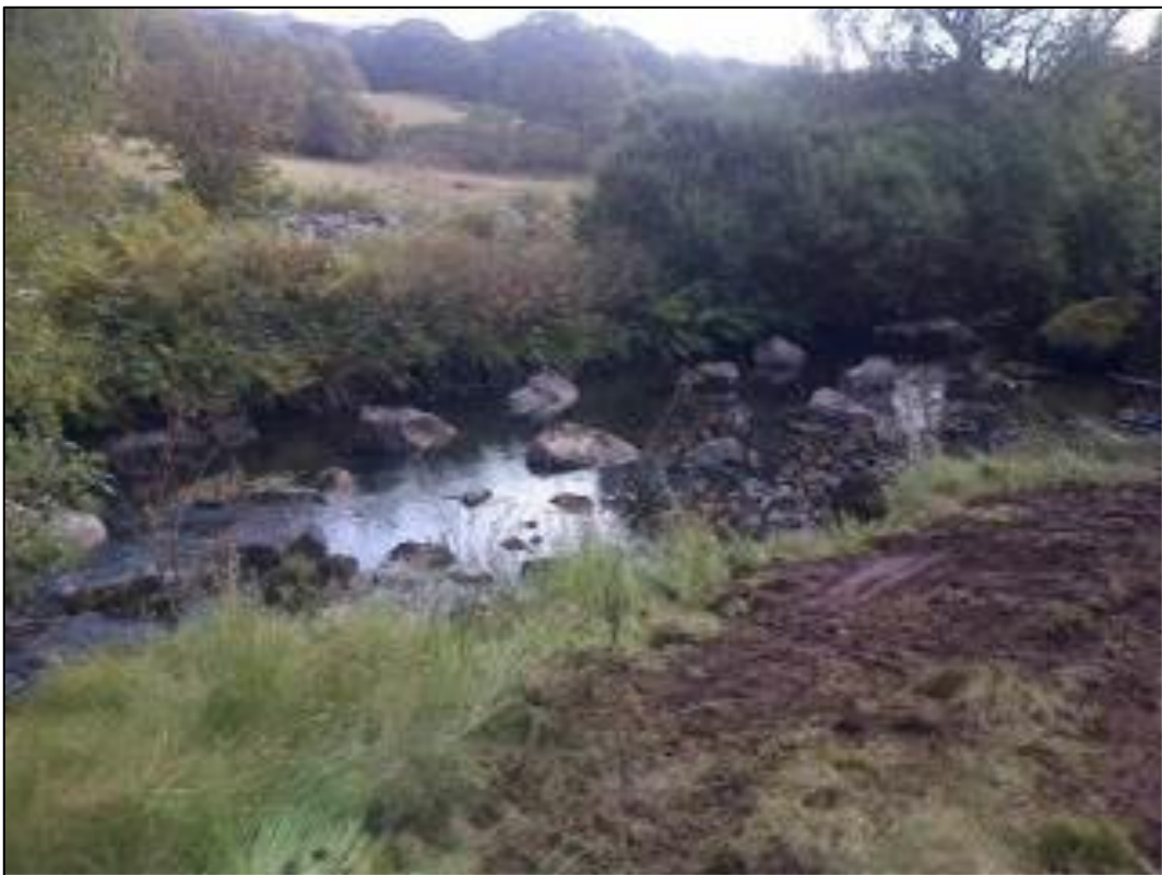
Boulder placement – After
