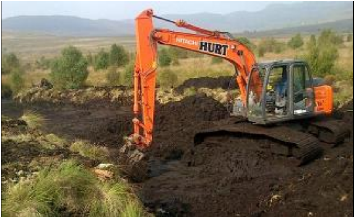
Settlement pond construction underway
