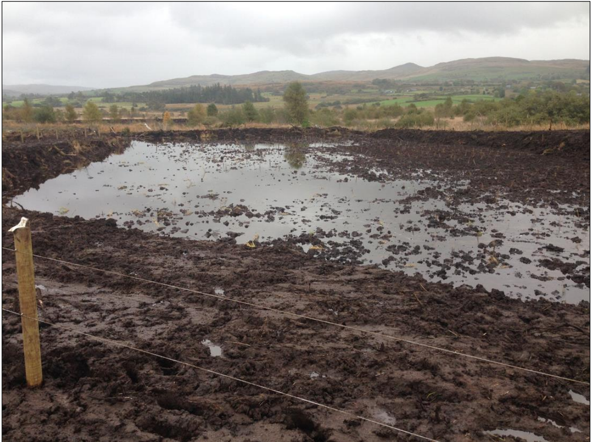
Settlement pond – immediately following construction
