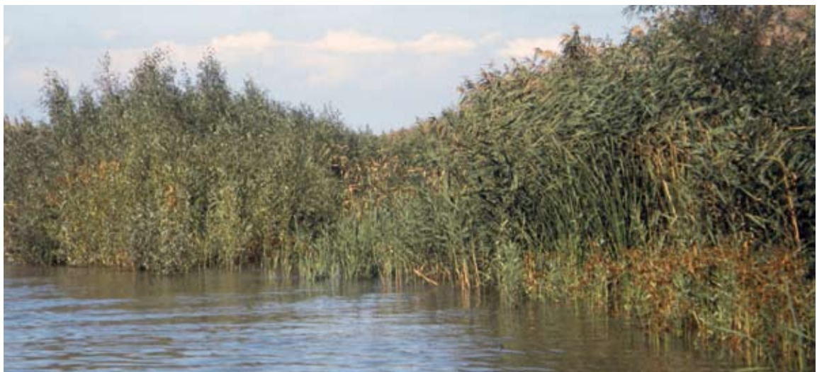
Fig. 27: The Babina main inlet canal (CC1), partially clogged by reed vegetation developed on new sediment deposits (2001)
