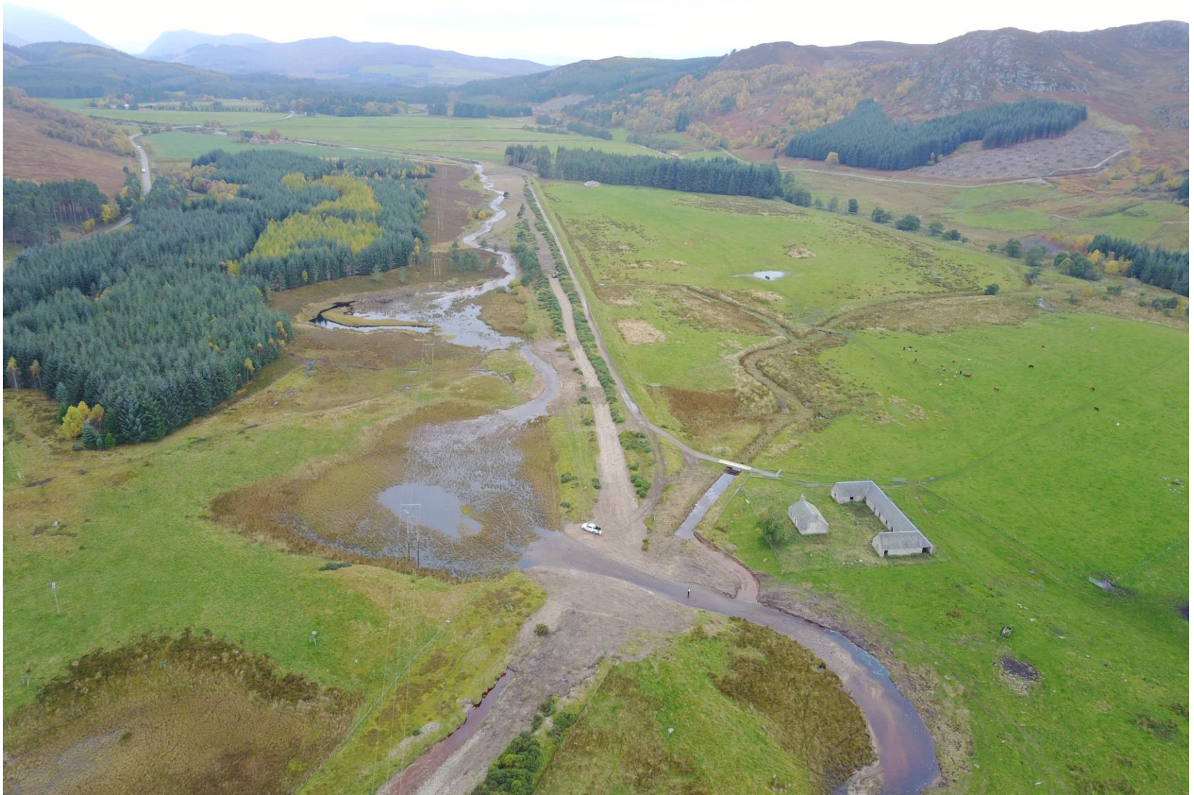
Aerial image of wetlands 2 and 1 (looking upstream) with previous canalised channel alignment still evident
