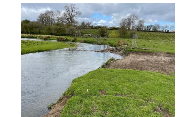
Lowered floodplain off take point with hinged tree downstream to encourage flow over floodplain.
