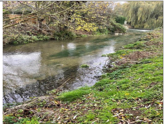
Newly installed brushwood berm in foreground (Queen Elizabeth Park)
