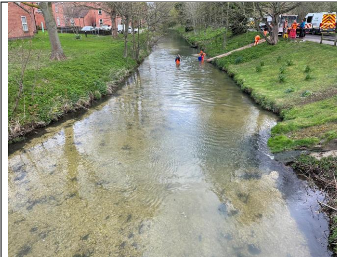
Limestone Gravel being added to channel in Stone Bridge Close Section.
