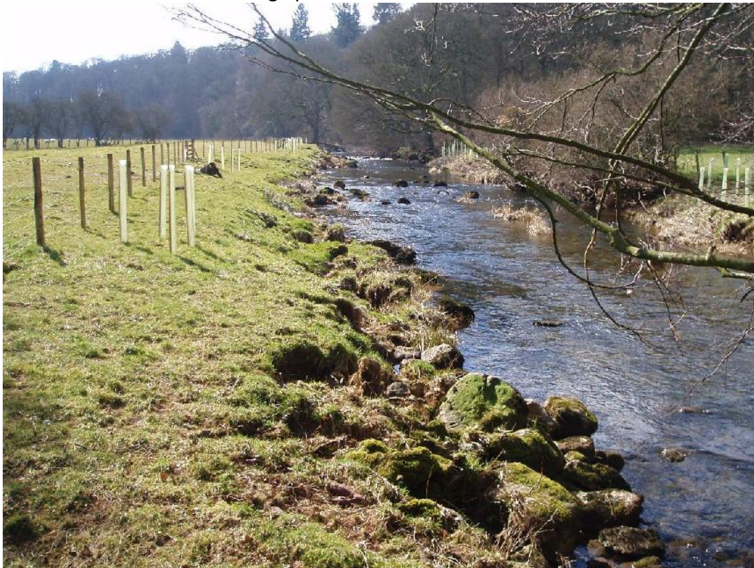
Picture 3. After work – looking upstream - March 2013. NY 61062 23745
