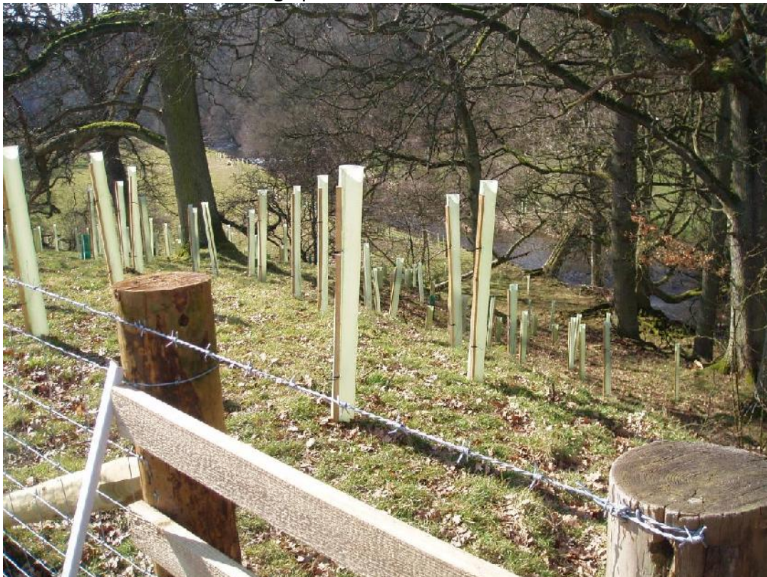
Picture 1. After work – looking upstream - March 2013. NY61096 23788.
