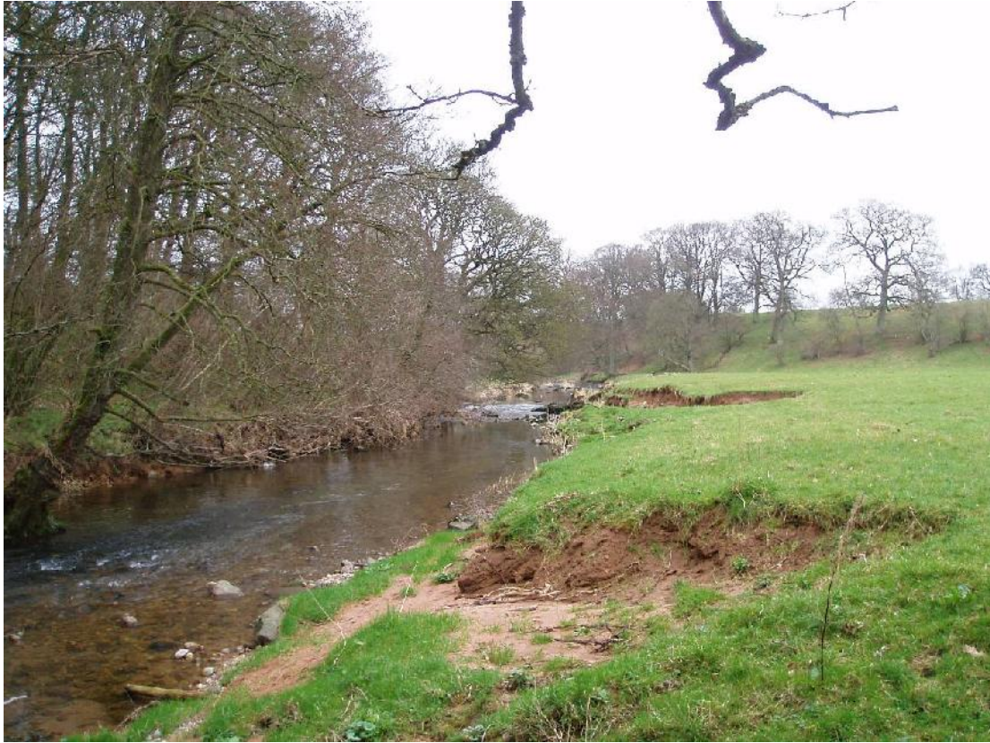
Picture 5. Before work – looking downstream – November 2012. NY61038 23583.
