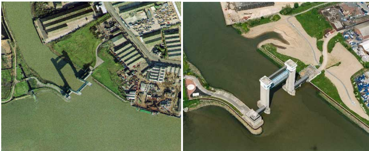
Figure 3.2: Creekmouth: before landscaping and flood defence improvement works, and after retreat of flood defence, construction of tidal backwater and landscaping works (EA Archive).
