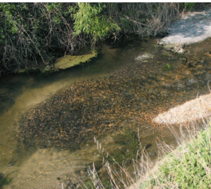
Creation of a riffle on the Couasnon at Vieil-Baugé
