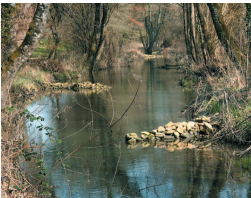
Flow deflector on the Couasnon
