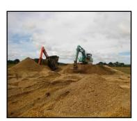
The top soil was removed and piled up. The first gravel layer was also removed and piled up ready to be returned to the hole at the end. This layer despite having gravels was also high in sands and silts. The second gravel layer found was considered a much purer layer and this was dug (up to several metres) and screened and stored ready to deposit into the dredged channel reaches.
