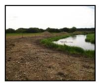
Despite grading and cleaning on site not all the fin silts and sands could be excluded from entering the river. However it was considered more effective than attempting to clean the gravels form the embankment.
