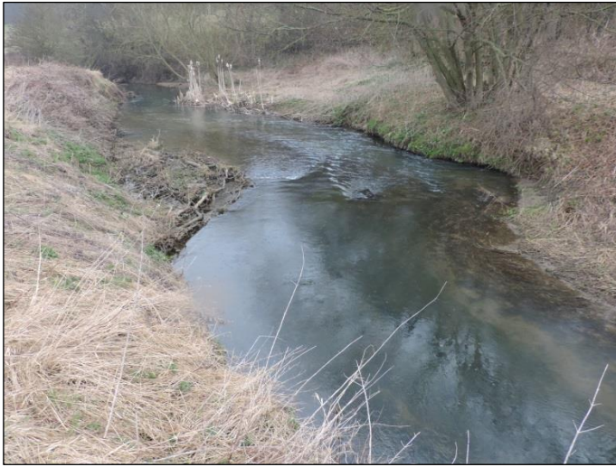
Fig 5. A brushwood mattress narrowing an over-wide riffle to promote natural cleansing of the gravels (Barkston)
