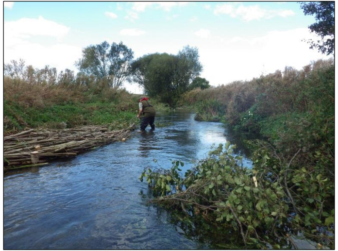
Fig 6. Completing a faggot mattress. (Syston)
