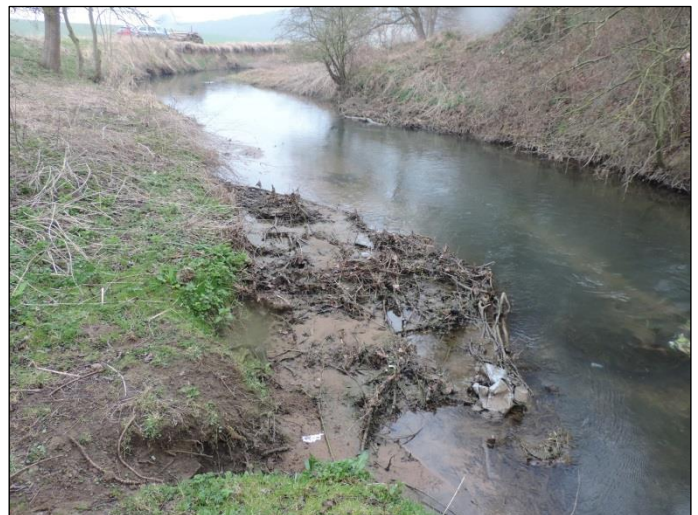
Fig 4. Open Brushwood mattress demonstrating the ability of these structures to trap large quantities of fine sediment. (Barkston)
