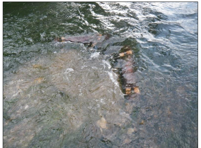
Fig 8. Paired micro-vanes, showing their ability to scour and clean gravel. (Syston)
