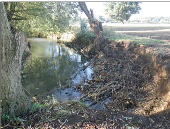
Fig 3. Erosion protection with an extensive log-faced brushwood mattress. (Syston)
