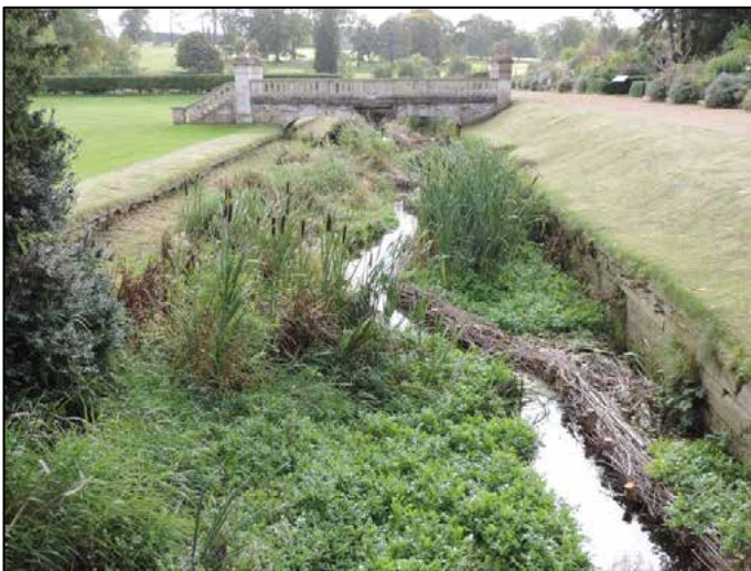
Fig 8. Narrowing using faggots infilled with brash and silt in the Walled Garden section (above before, below after). (Phase 1)
