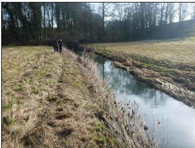
Fig 7. Channel narrowing using infilled brushwood mattresses, (a) before and (b) after. The right bank was reprofiled to create a 2-stage channel and excavated material was used to cover the adjacent brushwood mattresses and seeded. (Phase 1)
