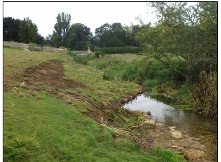
Fig 13. (a) The 2-stage channel creation in progress and (b) the completed works, which include turf-filled faggot-faced enclosures, prior to fencing being erected at the top of the reprofiled slopes. (Phase 1)
