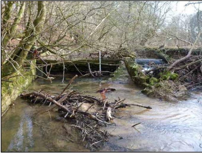
Fig 22. Upstream view of the weir (February 2013).
