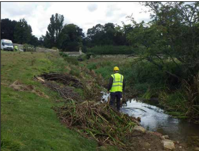
Fig 13. (a) The 2-stage channel creation in progress and (b) the completed works, which include turf-filled faggot-faced enclosures, prior to fencing being erected at the top of the reprofiled slopes. (Phase 1)
