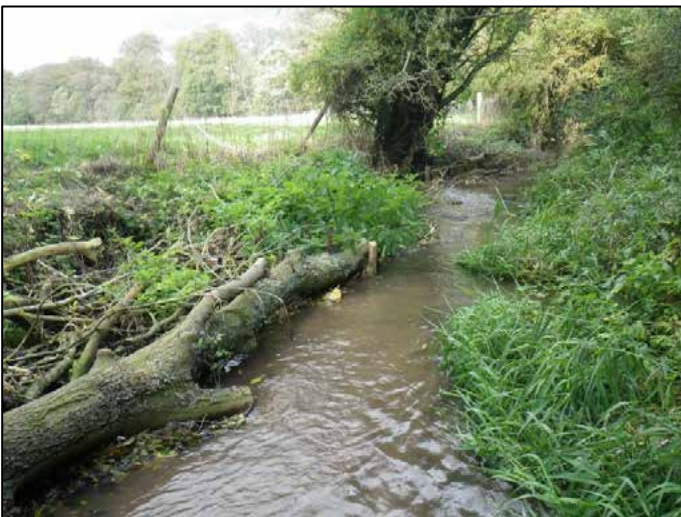
Fig 3. Riverside tree felled into the channel and secured with wire bindings. (Phase 2)
