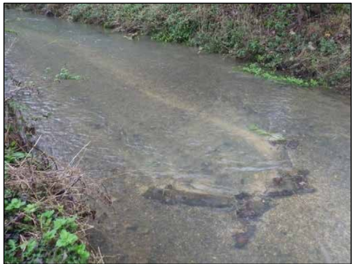
Fig 17. A single log flow deflector. (Phase 1)
