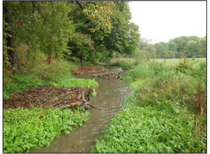
Fig 12. A series of log-fronted brushwood mattresses creating a narrower, more sinuous channel. (Phase2)
