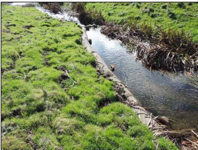
Fig 9. Log-faced enclosure infilled with earth and turfs. (Phase1) Fig 10. Log-faced brushwood mattress. (Phase2)
