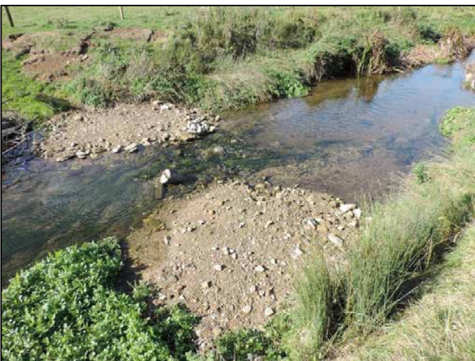
Fig 19. New pools showing the locations of excavated material which narrows the channel and encourages scour. (Phase 1)
