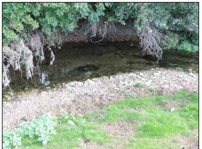
Fig 19. New pools showing the locations of excavated material which narrows the channel and encourages scour. (Phase 1)
