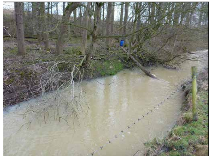
Fig 4. Felled tree and brush flow deflectors extending from high on the bank and secured by hooking around or wedging between multi-stemmed riverside trees. (Phase 3)
