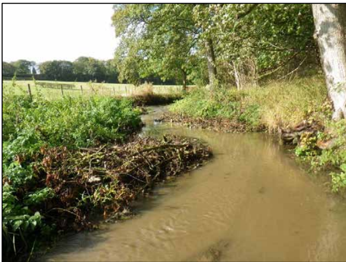
Fig 5. A series of offset brushwood mattress creating a narrow, sinuous channel. (Phase 2)
