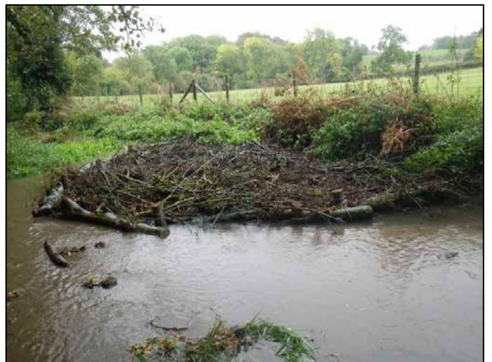
Fig 9. Log-faced enclosure infilled with earth and turfs. (Phase1) Fig 10. Log-faced brushwood mattress. (Phase2)
