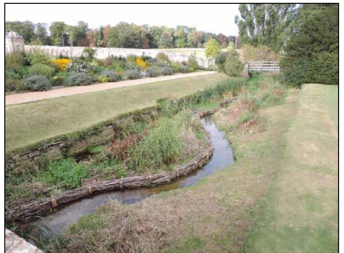
Fig 8. Narrowing using faggots infilled with brash and silt in the Walled Garden section (above before, below after). (Phase 1)
