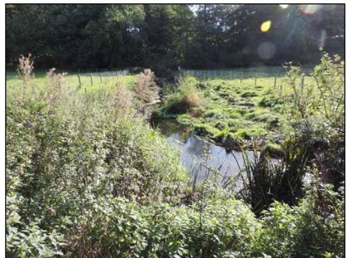
Fig 7. Channel narrowing using infilled brushwood mattresses, (a) before and (b) after. The right bank was reprofiled to create a 2-stage channel and excavated material was used to cover the adjacent brushwood mattresses and seeded. (Phase 1)
