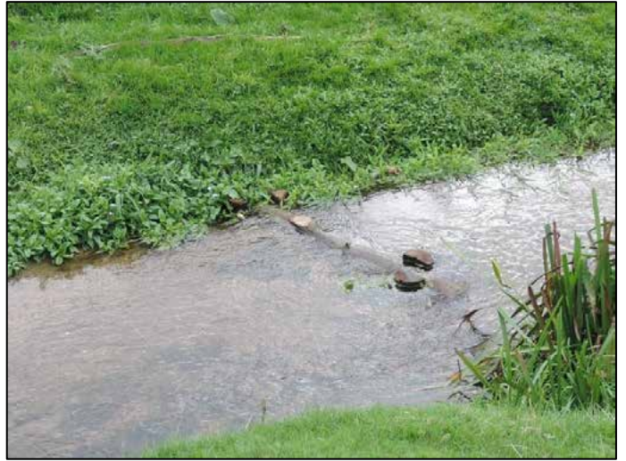
Fig 17. A single log flow deflector. (Phase 1)
