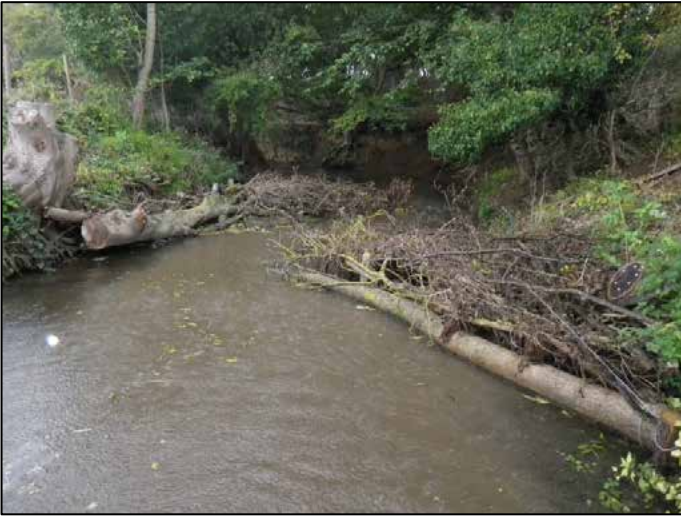
Fig 11. Offset log-fronted brushwood mattresses created by felling trees into the channel and infilling with brush. (Phase2)
