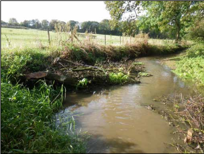
Fig 1. Hinged and pinned live sycamore. (Phase 2)
