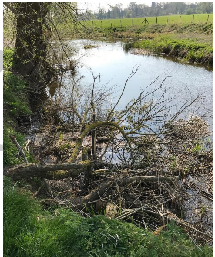
Figure 2 Hinging and pinning of a smaller tree at Ailsworth
