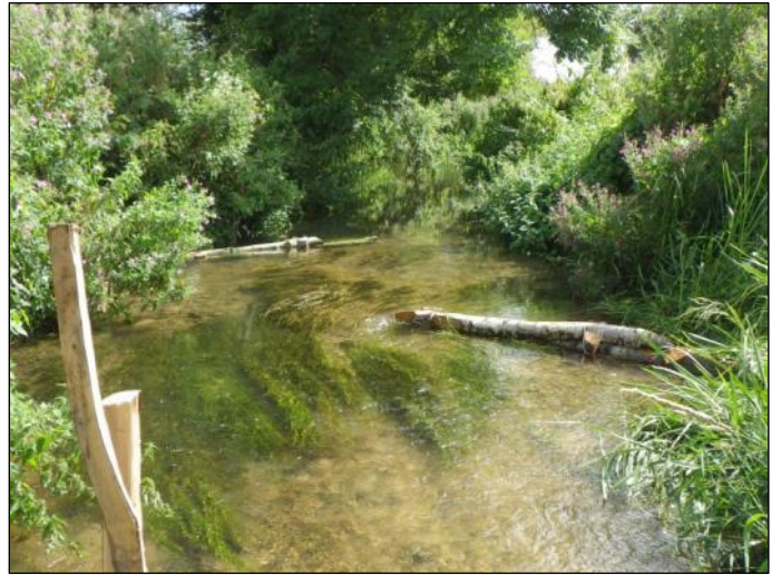
Fig 10. Off-set flow deflectors under construction (Phase 2)
