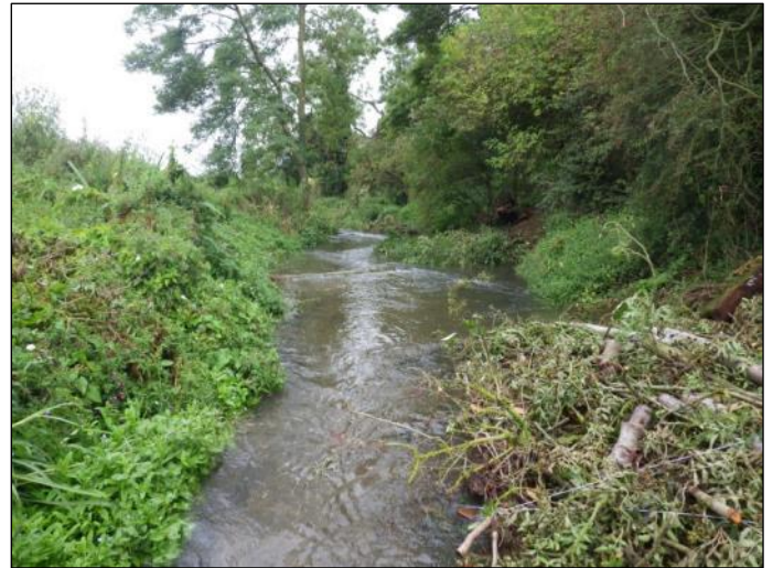
Fig 6. Open brushwood mattress (Phase 2)
