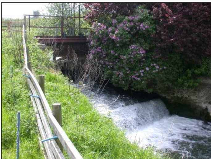
Fig 15. The sluice on the Great Ponton Mill bypass channel
