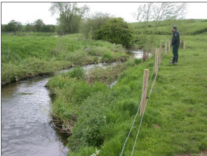
Fig 14. Riverside fencing protecting the marginal wetland vegetation and layered enclosures (Phase 1)
