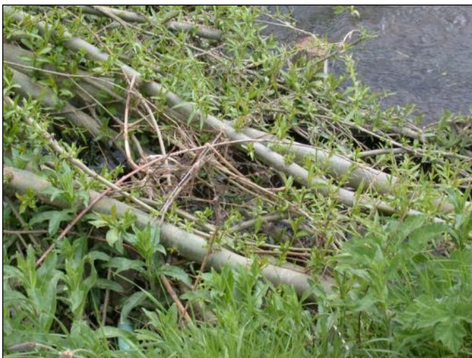
Fig 3. Willow layering detail (Phase 1)
