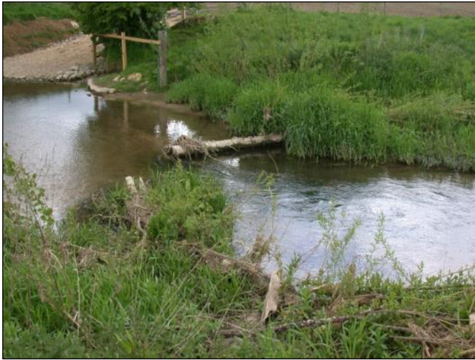
Fig 9. The paired flow deflectors below the ford installed by GAAFFS in 2008
