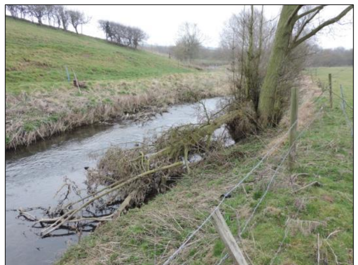
Fig 8. Hinged and secured alder following winter high flows (Phase 2)
