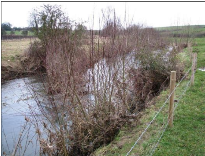
Fig 1. Regeneration of the live willow logs used by GAAFFS to narrow the channel in 2008
