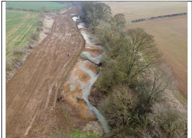
View of top section of site after works Credit: Andrew Chick
