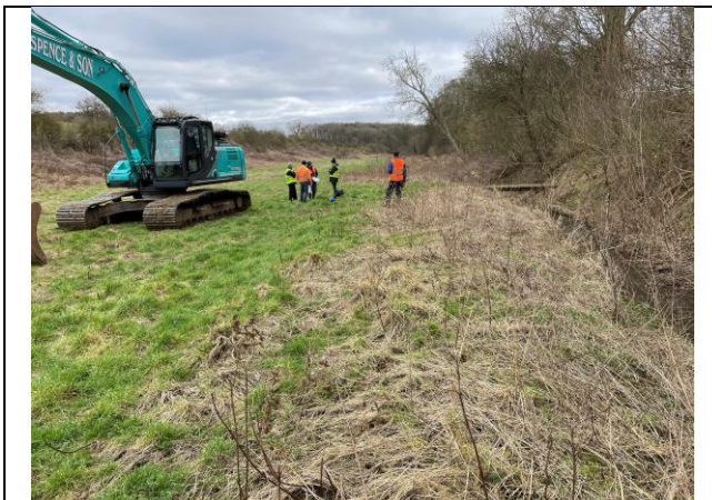
Site before works with old channel to right Credit: EA
