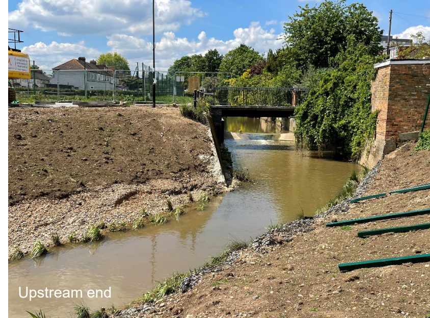
Old channel after backfilling
