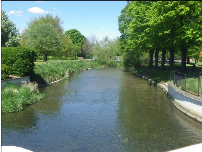
Fig 1. Before (May 2017). Looking downstream from White Bridge showing the original wide channel and concrete banks
