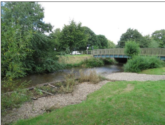
Fig 7. The eroded bank has been restored behind a faggot and gravel enclosure and planted-up with native plants. The willows behind have been coppiced or pollarded.
