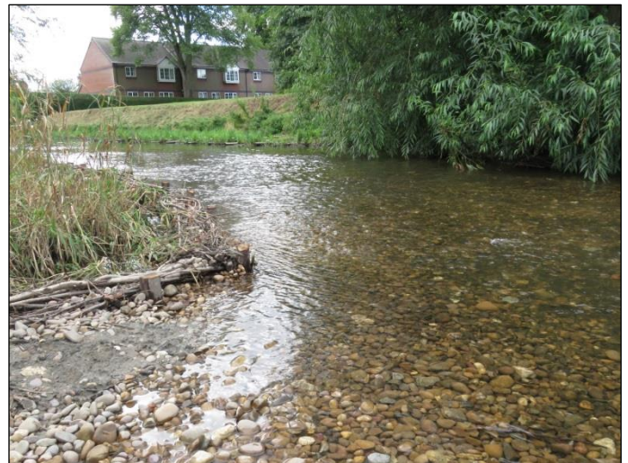
Fig 6. Fine sediment excavated from the bed has been replaced with fresh, clean gravel.
