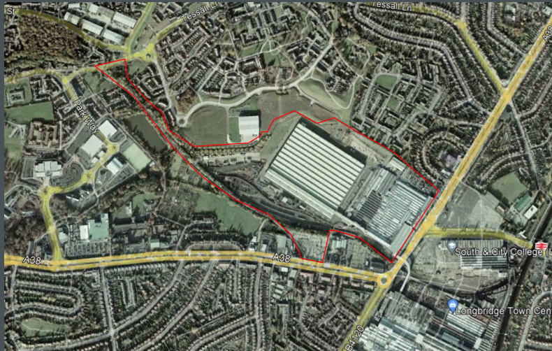
Pre-demolition Longbridge West Site – River Rea culverted under railway serving former factory
