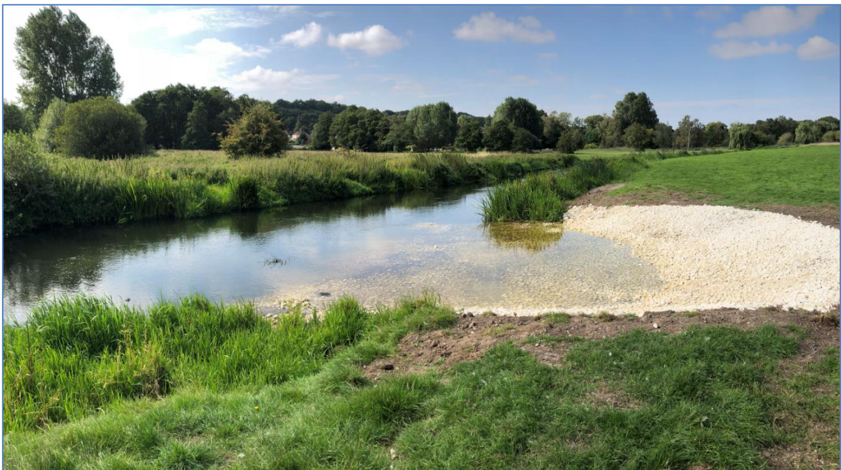
Imported chalk used to create hard surface to reduce sediment input from cattle poaching. The shallow warm water will provide a fry refuge habitat.
