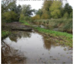
Image: Removal of spoil embankments at selected locations has restored the connection between river and floodplain during high flows
