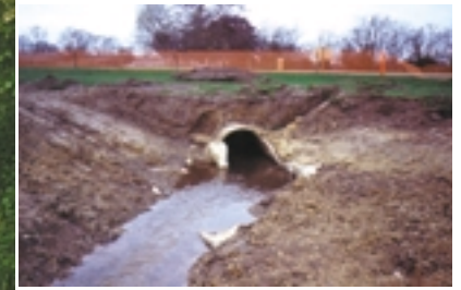
'Daylighting' of the Ravensbourne
