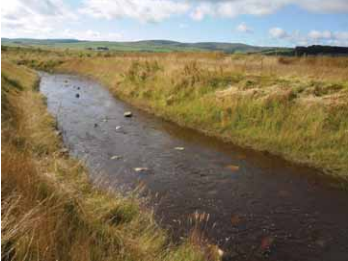
August 2012 – Day of Tie-In (View looking south from southern bank)
