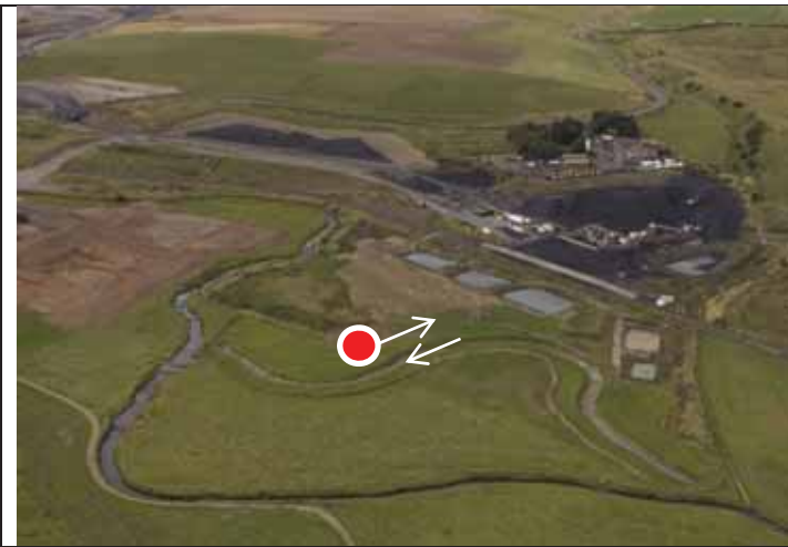
September 2011 – Construction Complete
