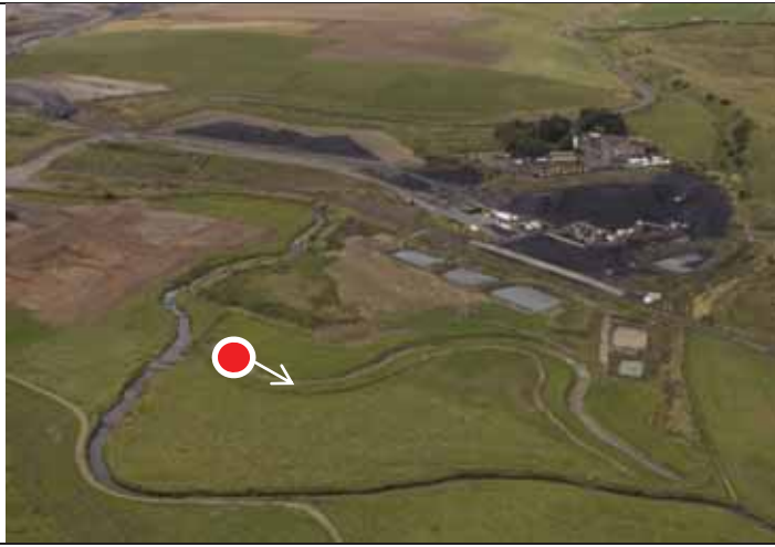
September 2011 – Construction Complete
