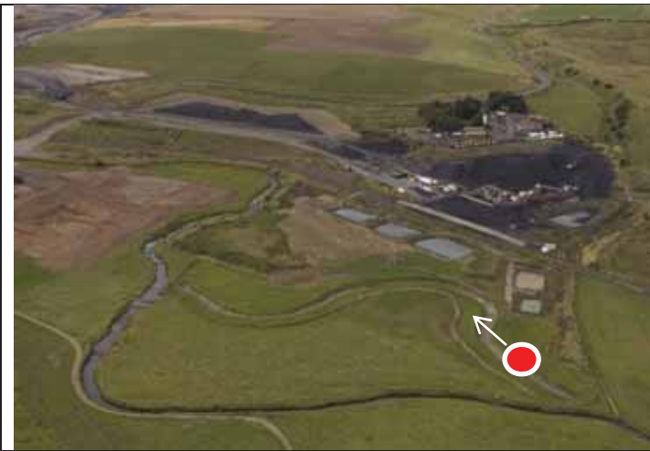
September 2011 – Construction Complete
