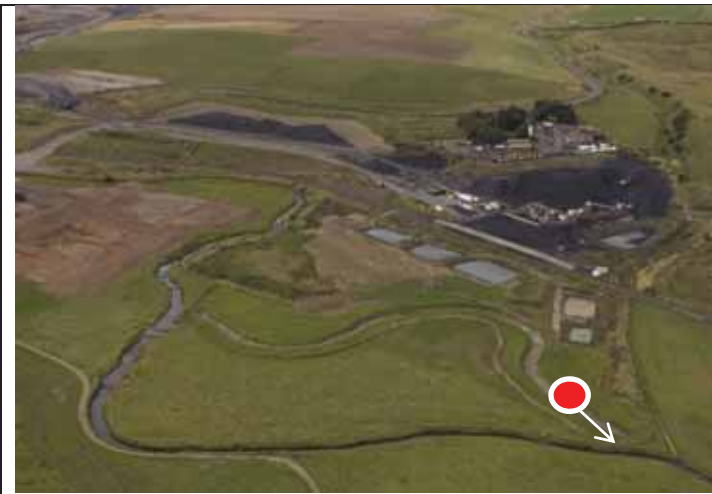
September 2011 – Construction Complete
