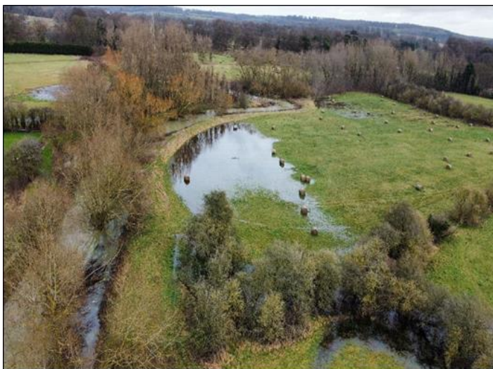
Fig 3. The presence of the historic floodbanks are counter productive for land drainage and improvement. The floodbanks might protect floodplain from inundation from river but trap surface water run off behind the banks reducing drainage of land. The Witham is a ground water fed river which naturally has a high water table and despite considerable effort to drain this landscape through deepening of river and flood banks has not achieved aims of improving agricultural yields and has left the river unable to recover ecologically without significant intervention,
