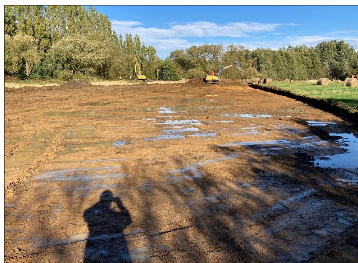
Fig 7. Two stage floodplain with a lowered inset floodplain that will inundate more frequently and then the un lowered floodplain with grass still present to right of image. In places the floodplain was predominantly clay and scrapes were installed over the impermeable geology.
