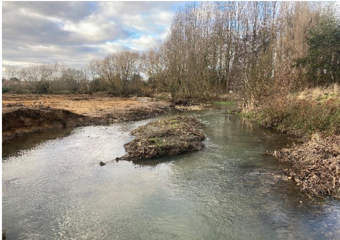
Fig 11 The shows difference in height of historic embankment and of the newly lowered inset floodplain to illustrate what a well-connected floodplain should look like. ,
