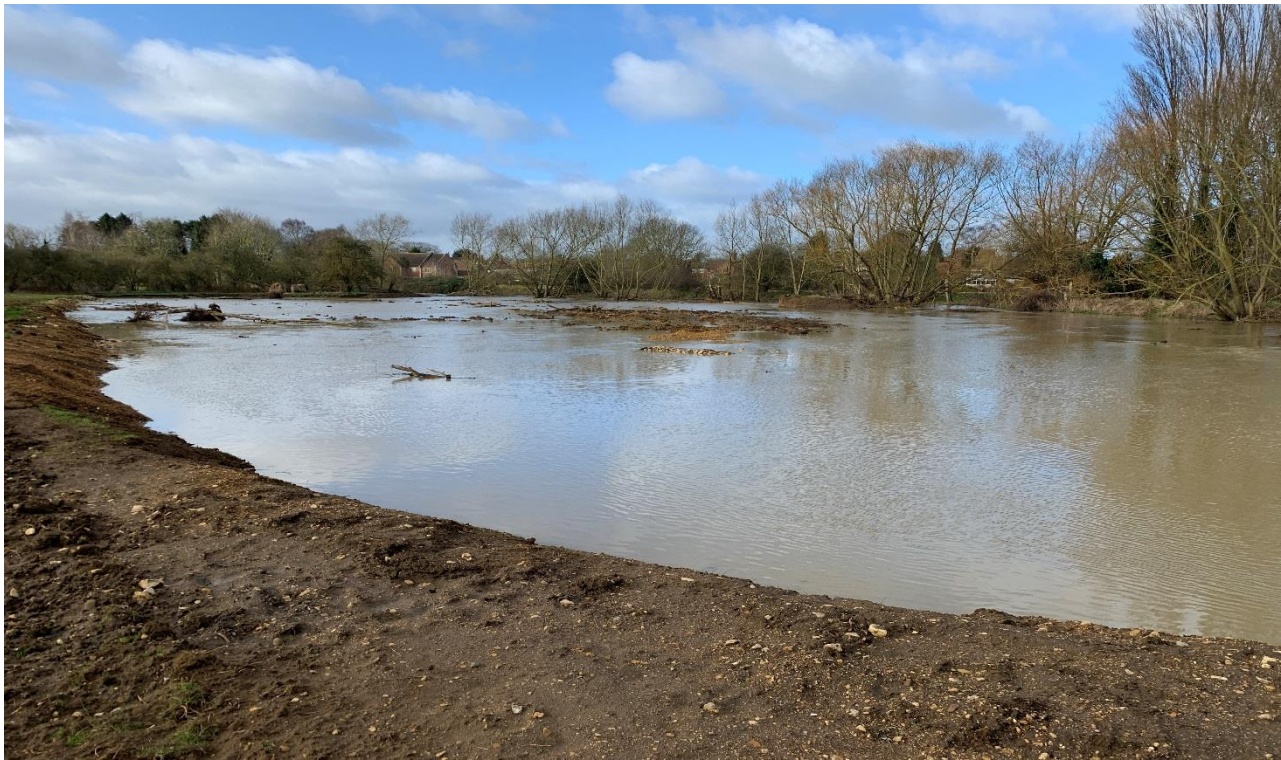
Fig 11 The shows difference in height of historic embankment and of the newly lowered inset floodplain to illustrate what a well-connected floodplain should look like. ,
