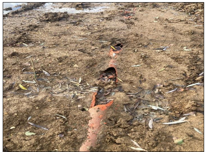
Fig 6. Modern historic land drains uncovered during floodplain lowering to try to drain and improve unsuitable heavy clay soils for agriculture.
