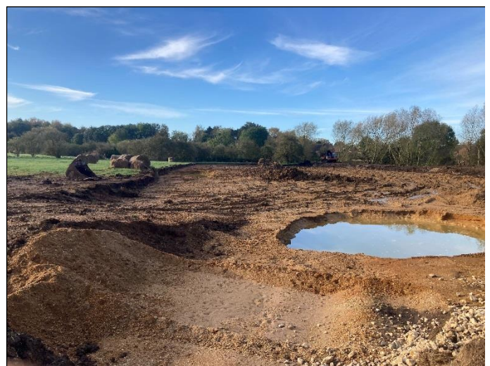
Fig 8. Floodplain ponds and scrapes added to create habitat diversity. Floodplain and top of valley where spoil was spread has been reseeded with native wildflower mixes to maximise benefits for pollinators and biodiversity.
