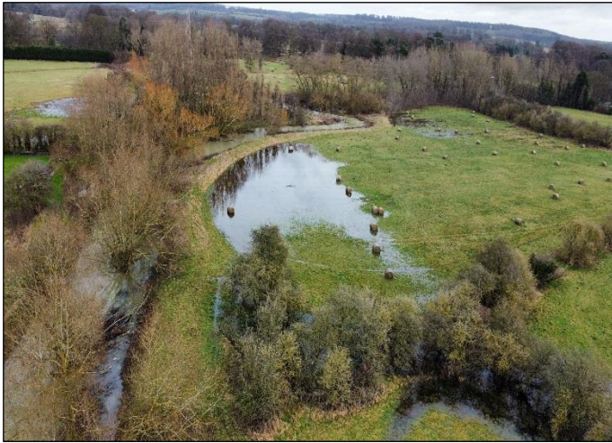
Fig 1. Before (Feb 2021). High water event and heavy rain had caused the Witham to come out of bank further downstream overtopping defences – at Manthorpe flood water didn't occupy the floodplain but instead the defences prevented surface water draining into the Witham
