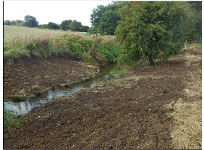
Fig 7. Sections of 2 stage channel created by reprofiling the bank against a new (a) faggot and (b) log bank toe.
