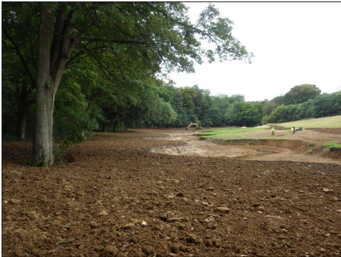
Fig 20. Reprofiling the excavated soils
