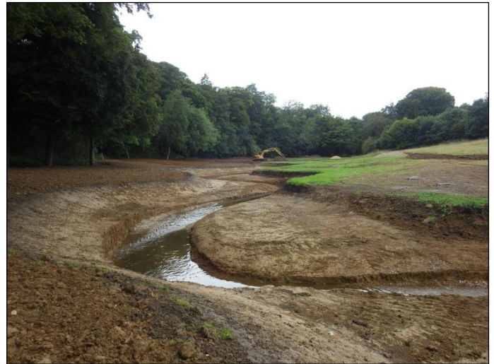
Fig 21. The completed scheme
