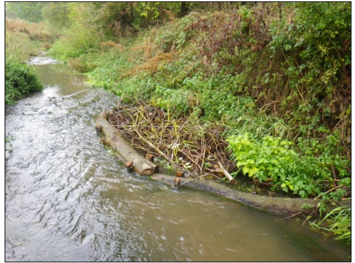
Fig 4. Completed log-faced brushwood mattress
