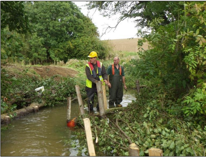
Fig 3. Log-faced brushwood mattress under construction
