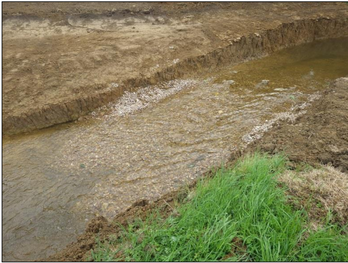
Fig 18. One of the new riffles
