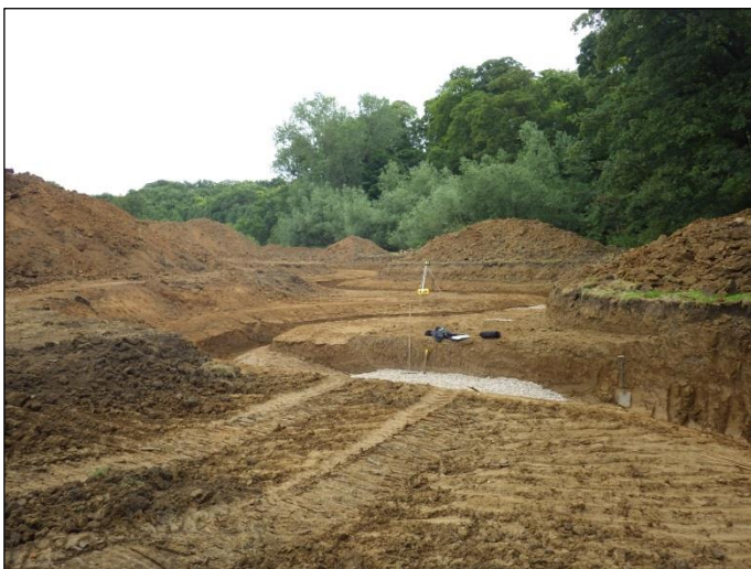
Fig 16. The meanders and berms are taking shape
