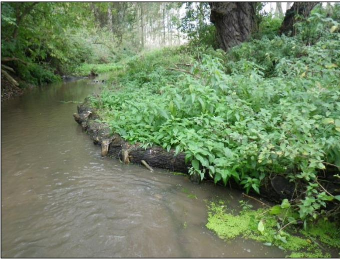
Fig 8. New berm stabilised by vegetation.
