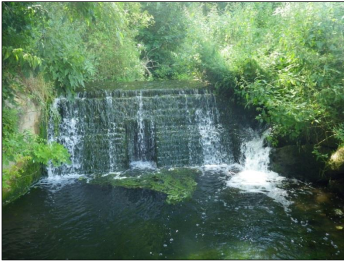
Fig 11. Grange Farm Weir
