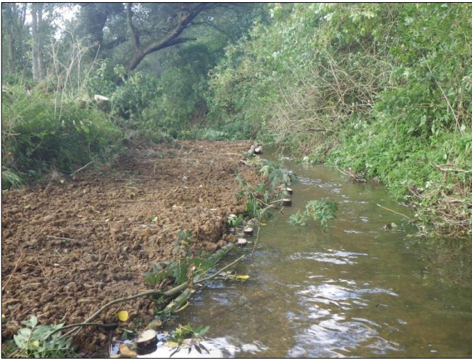
Fig 7. Sections of 2 stage channel created by reprofiling the bank against a new (a) faggot and (b) log bank toe.
