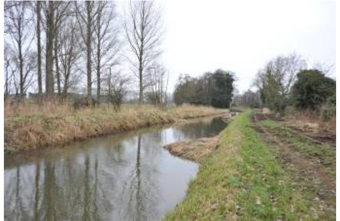
Nar Narborough – ‘Pools’ 9 & 10 plus shoulder formed over old deflector – soft peat shoulders with reeds; indistinct deepening – non-existent pools (looking d/s with pool 11 in background)
