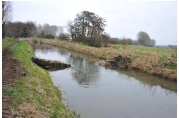
Nar Narborough – Non-existent ‘Pool’ 13 plus shoulder formed over old deflectors – very soft peat shoulders with limited reeds – looking u/s
