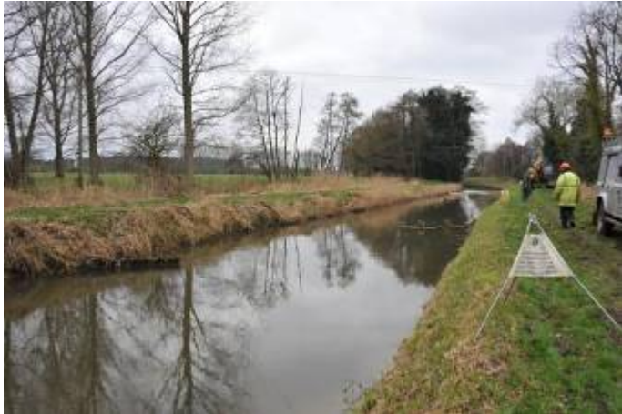
Nar Narborough – ‘Pools’ 9 & 10 plus shoulder formed over old deflector – soft peat shoulders with reeds; indistinct deepening – non-existent pools (looking d/s with pool 11 in background)
