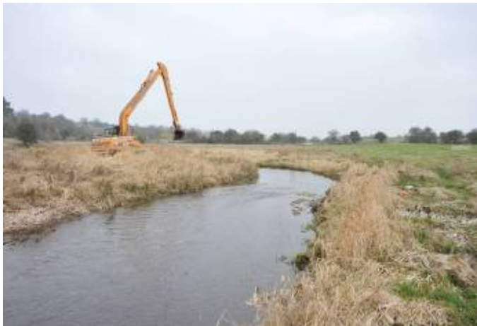
Nar Castle Acre – narrowing and shallow run/riffle formation (Photo ref: CA9)
