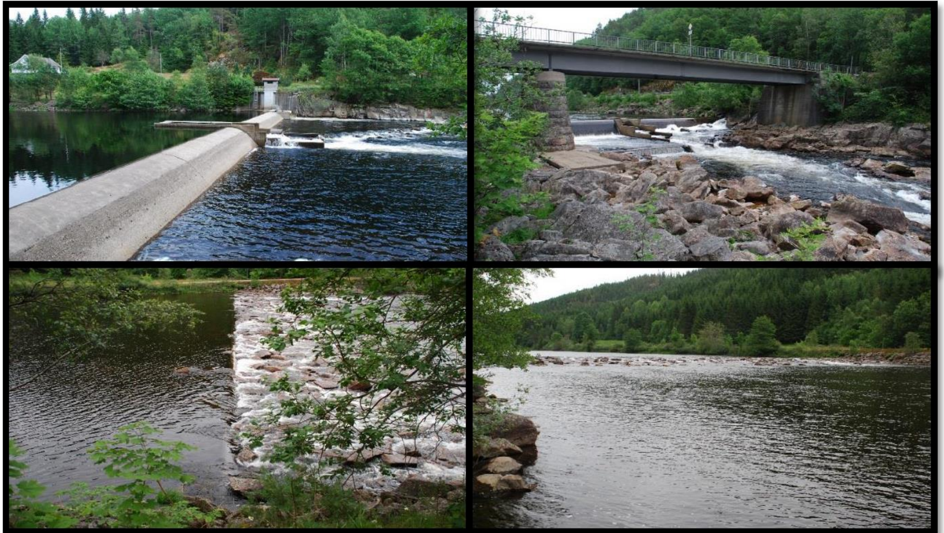
Figure 7. Weirs in Laudal bypass section (Mandalselva River). On the upper left corner Manflå Dam, upper right corner Kleveland concrete weir, both on the bottom are one of the 9 cobbles weirs view from two sides. Photos: Berit Köhler and Ana Adeva.
