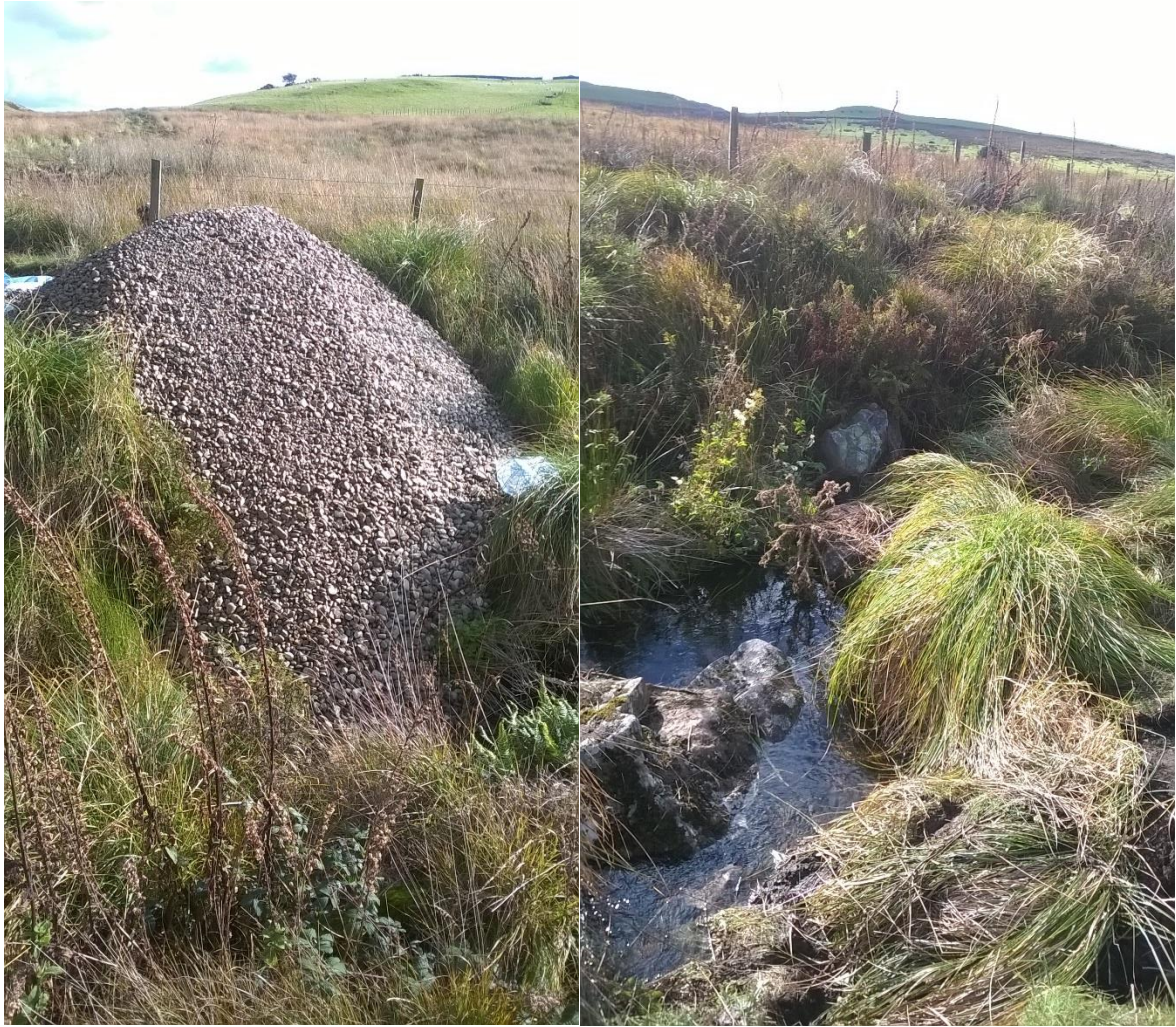
Lower gravel stockpile at the start of the higher gradient section. This gravel is expected to be dispersed more quickly than the upper stockpile. Boulders placed in the river were originally removed from the channel in 1995-6.
