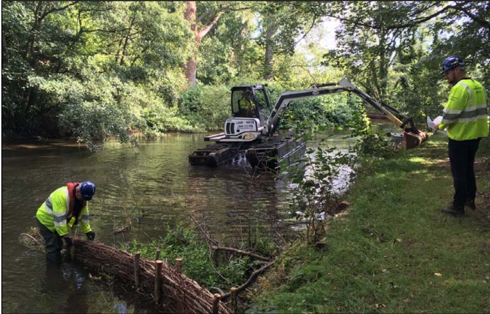
Amphibious excavator re-profiling bank profile.
