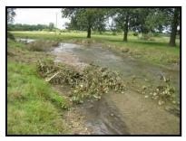
In locations where the limbs were to be used in channel, trenches in the bank were dug with at least a third of the limbs length buried providing a secure structure. In this reach high concentrations of gravel within the bed stopped the normal technique of using wooden stakes from being used.
